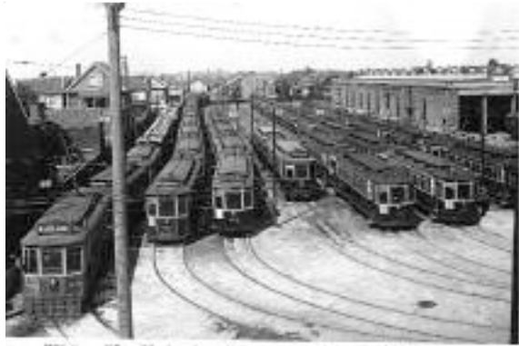
8866. St. Clair Car House, looking W. (2), July 10/24
